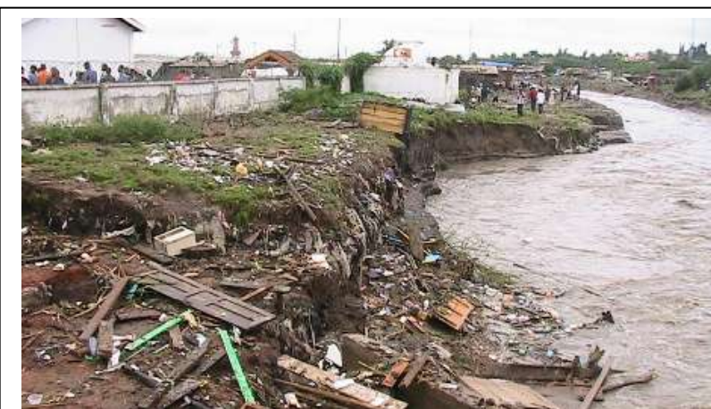
July 2010 floods: Storm drain at Jerico, Ashaiman
